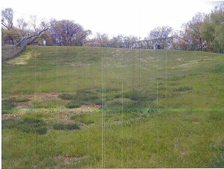
Looking upstream at the downstream slope of the dam embankment.
