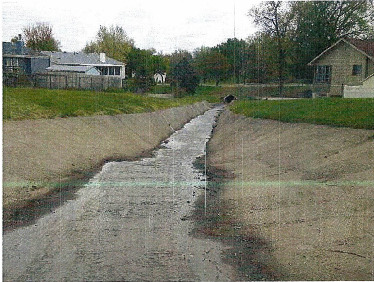
Looking downstream along the spillway.
