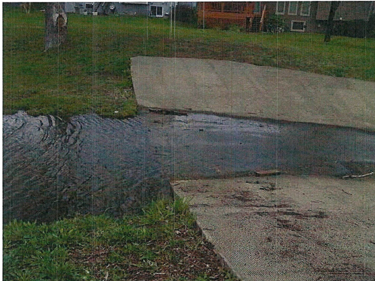
The spillway inlet.
